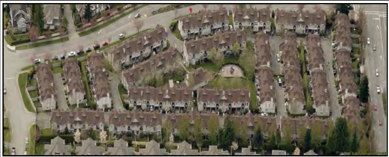
Willow Arbour Condominiums LMS192 – 8716 Walnut Grove Drive, Langley, BC – 2009 $600,000 Cedar Conversion Contact person: Glen Mason – Property Manager – Strataco Management Phone number: 604.294.4141
