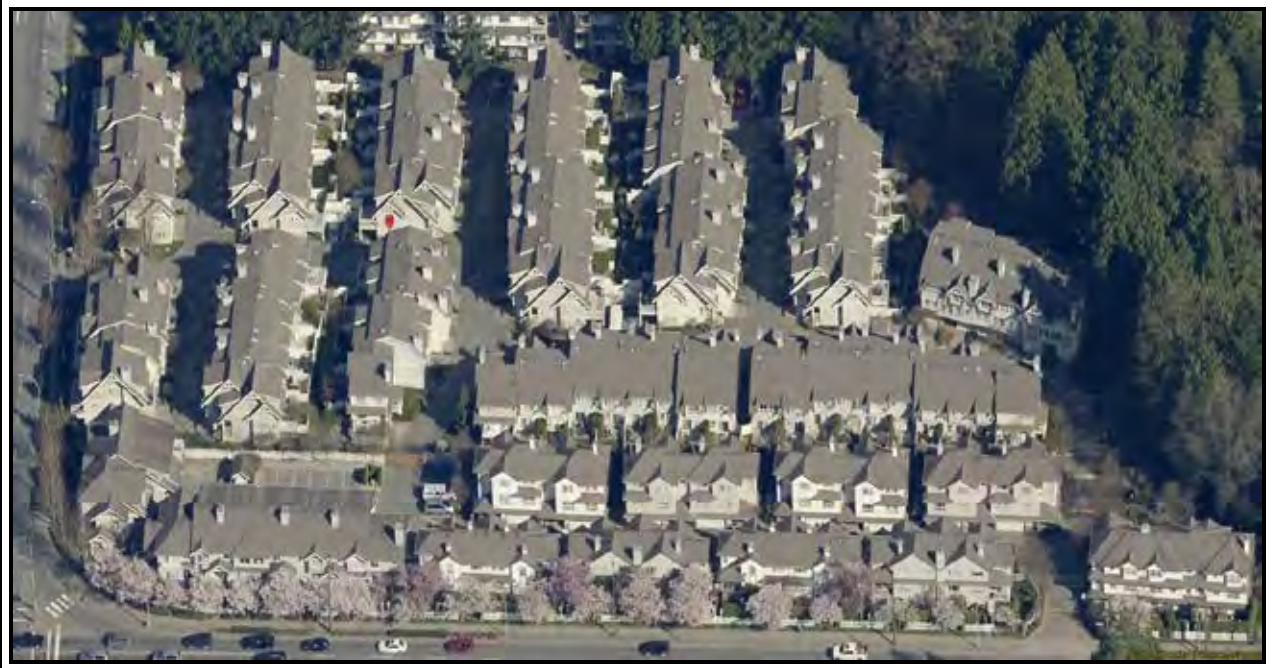
Mayberry Condominiums LMS2706 – 8844 208 th Street Langley, BC -2009 $600,000 Shingle to Shingle Contact person: Brian Belfour – Property Manager – Baywest Phone number: 604.595.8645
