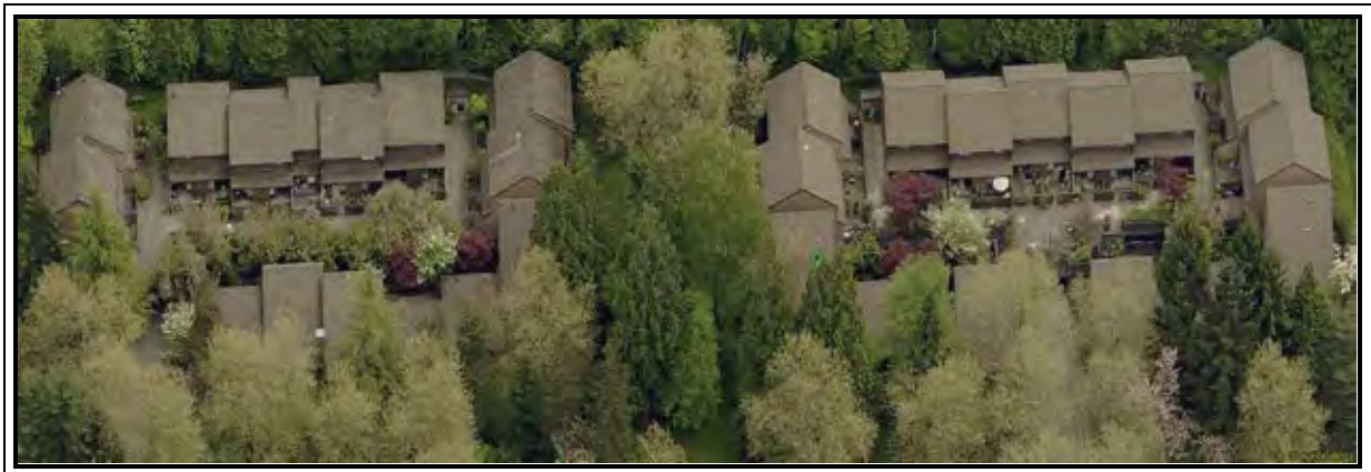
Garden Grove NW 603 – 4102-4396 Garden Grove Drive Burnaby - 2015 $215,000 Shingle to Shingle Contact person: Don Marsh roofing consultant Phone number: 604.435.0710
