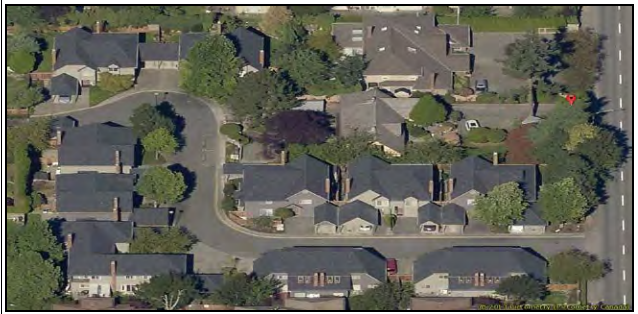
Empress Court Condominiums NWS2065 - 8631 No.3 Road, Richmond – 2011 $200,000 Cedar Conversion Contact person: Laurie Evens – Property Manager, Century 21 Phone number: 604.273.1745
